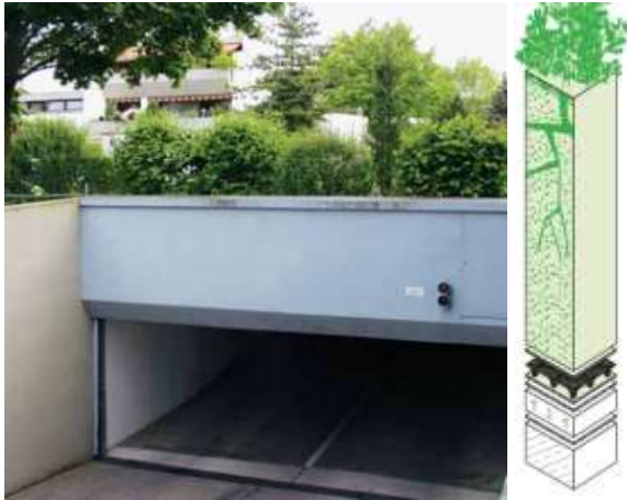
Fig. 6. Composition of a Ground Level Green Roof [6].
