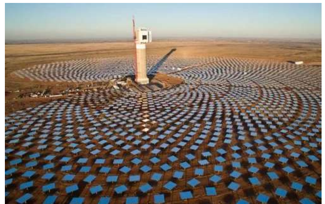
Fig. 2. Central Tower Receivers for Solar Thermal Electricity [8]
