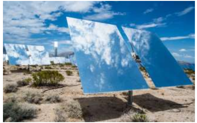
Fig. 1. Heliostat Field [4]
