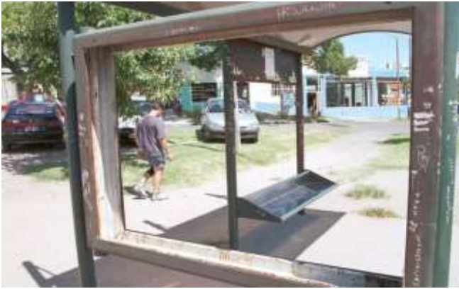
Fig 13. Stop in poor condition
