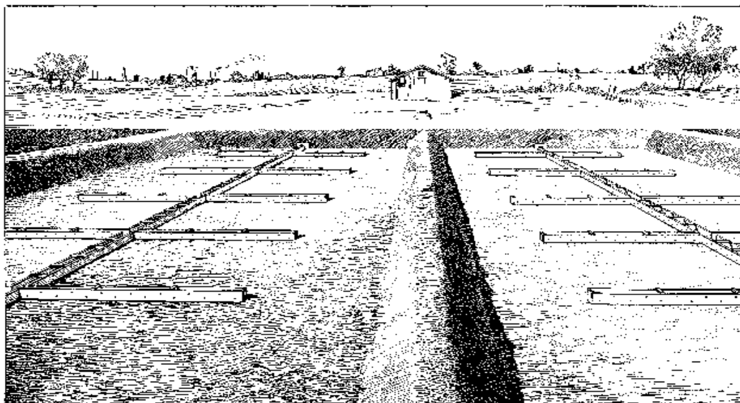
FIG. 133. DISTRIBUCION SYSTEM FOR INTERMITENT SAND FILTRATION.
