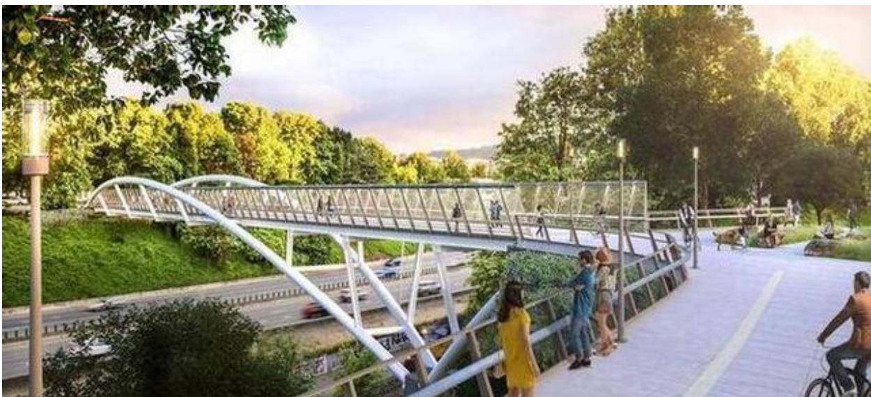
Figura 73. Puente para peatones y bicicletas de Earl Blumenauer. (Fuente: https://www.portland.gov/transportation/pbot-projects/construction/congressman-earl-blumenauer-bicycle-and-pedestrian-bridge ).
