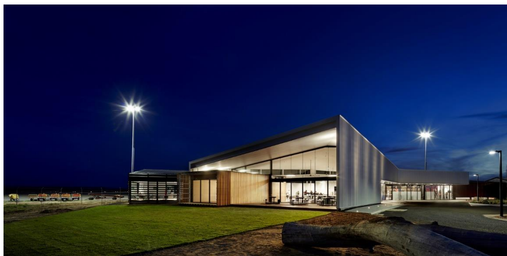
Figura 20 Terminal Aérea de la Isla Canguro, Australia – Vista exterior. Fuente: https://www.archdaily.com/911713/kangaroo-island-air-terminal-ashley-halliday?ad_medium=gallery
