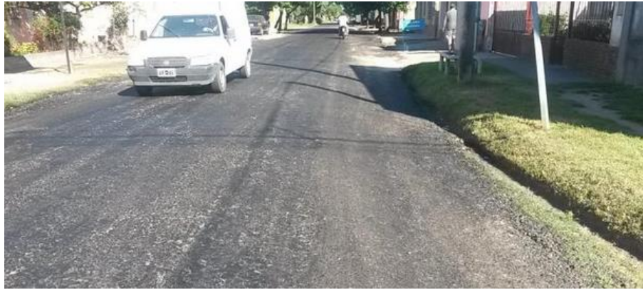
Figure 2. RAP use only in a suburban area in the Municipality of San Pedro (Buenos Aires, Argentina)
