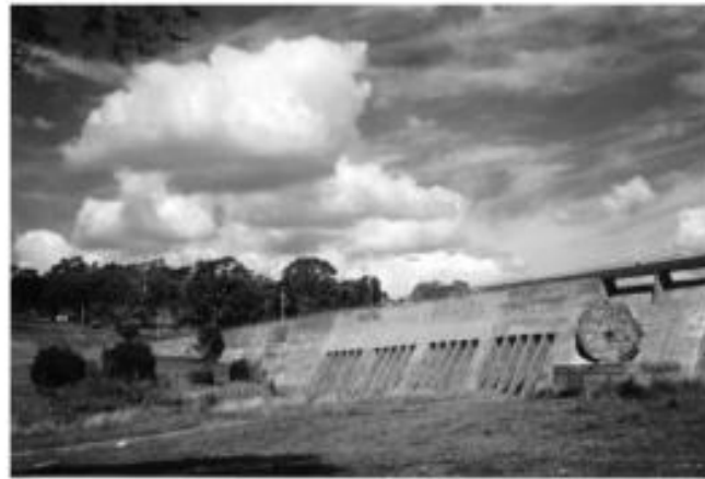
Figure 1. Tandil dam (Buenos Aires province, Argentina).
