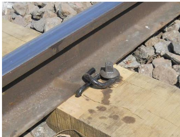
Figura 71: Gauge-Lock (Clip de Pandrol).
